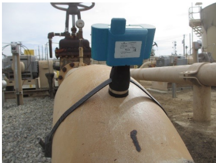
Ultrasonic sensor monitoring petroleum pipeline (Emerson)
